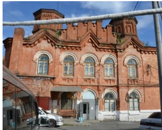
30. Achinsk synagogue, western façade
